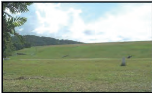
View of Existing Dam Embankment
