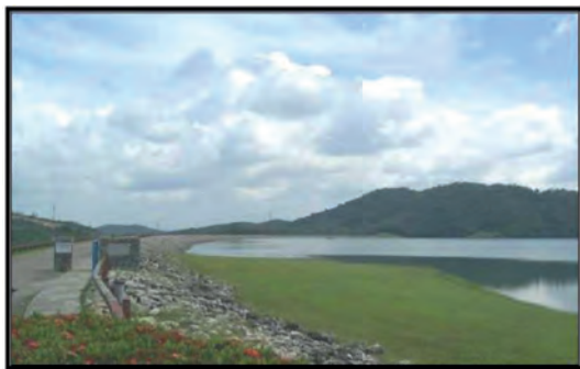
View of Existing Dam Crest
