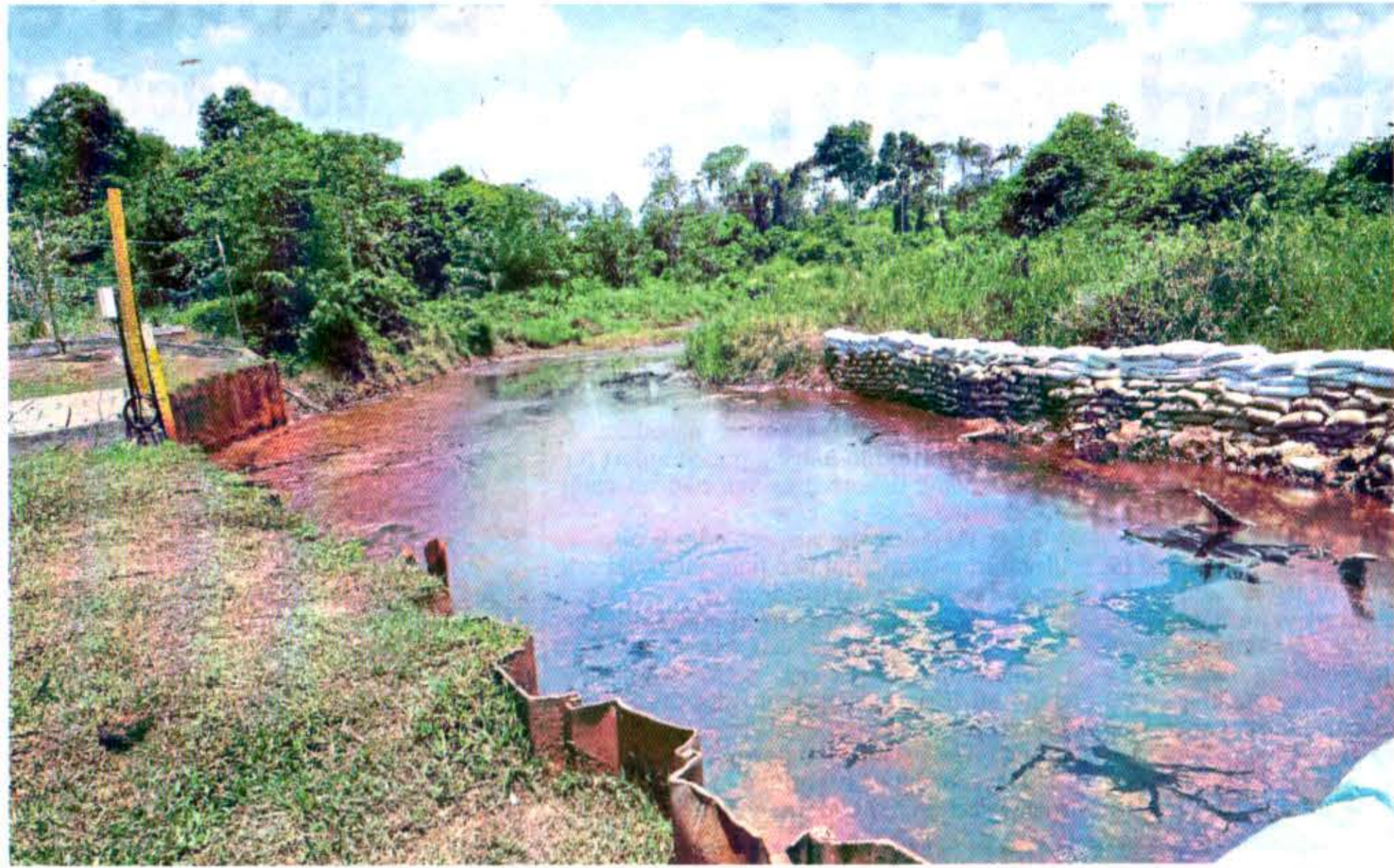
Critical: The low water level of Sungai Sedili Kecil at the Lok Heng water treatment plant.
