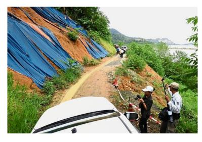
Preventive measure: Plastic sheets lining one of the 23 landslide sites in the Mengkuang Dam area.
