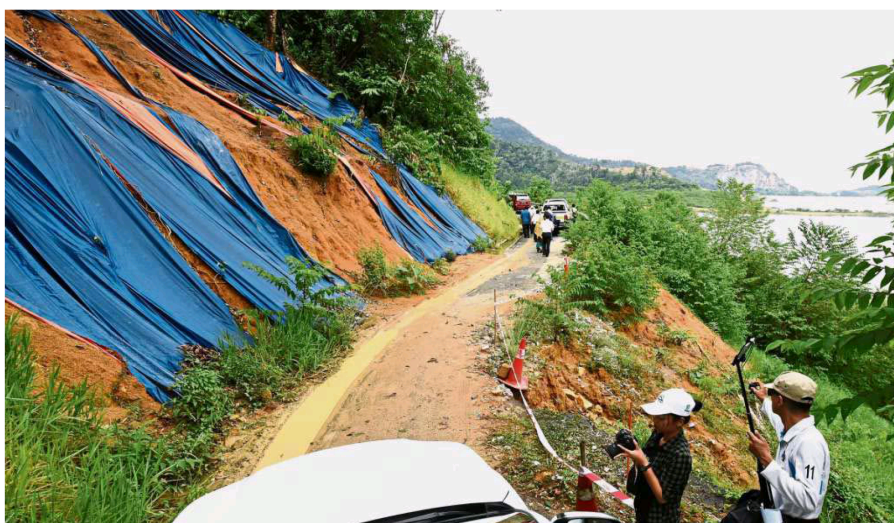
Preventive measure: Plastic sheets lining one of the 23 landslide sites in the Mengkuang Dam area.
