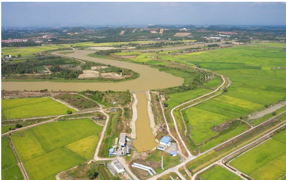
The Sungai Muda has dropped in water level at the Lahar Tiang intake.
