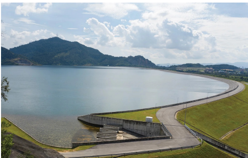
17.12.2021 : MENGGUANG DAM EFFECTIVE CAPACITY AT 93.9%
