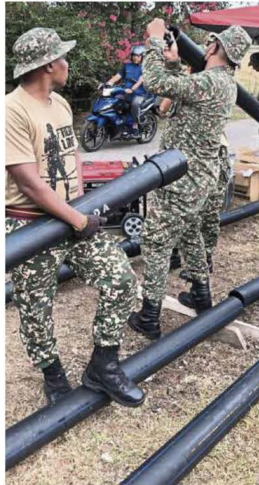
The team helping to lay pipes in Kedah.
