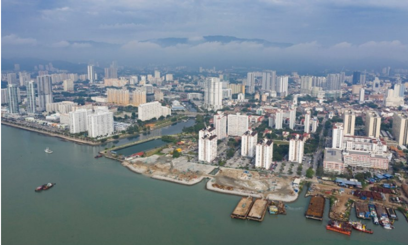
3rd Penang Twin Submarine Pipeline (3rd PTSP) project, Macallum Site
