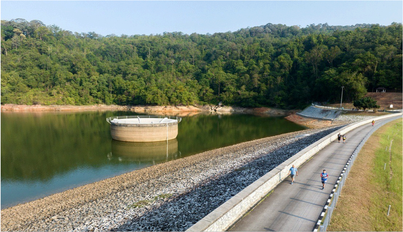
PBAPP AIR ITAM DAM AT 51.8% EFFECTIVE CAPACITY (10.4.2023)
