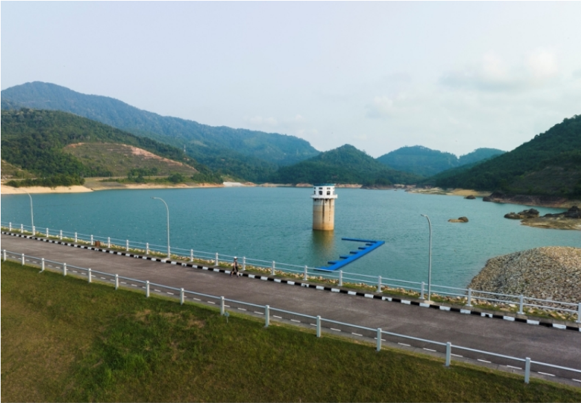
PBAPP TELUK BAHANG DAM AT 50.7% EFFECTIVE CAPACITY (13.4.2023)
