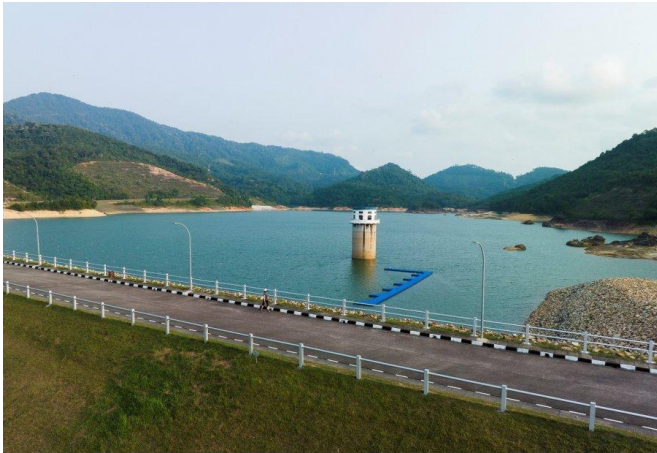
PBAPP TELUK BAHANG DAM AT 50.7% EFFECTIVE CAPACITY (13.4.2023)
