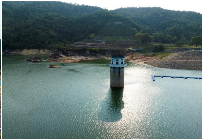
PBAPP TELUK BAHANG DAM AT 50.7% EFFECTIVE CAPACITY (13.4.2023)
