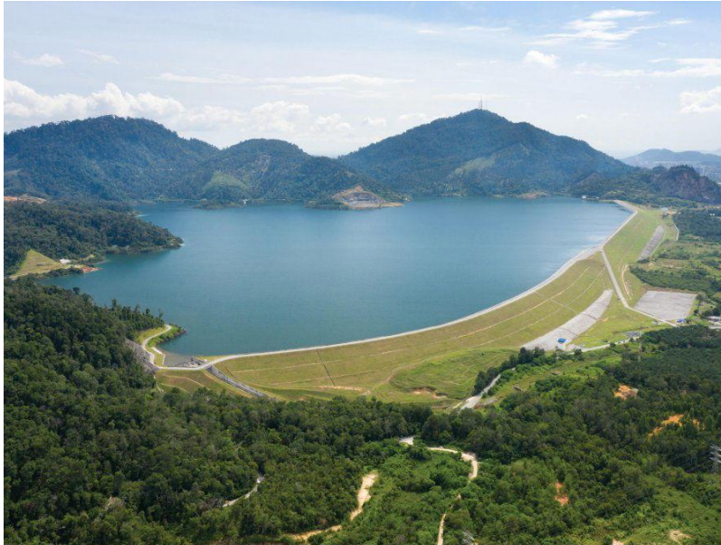
Expanded Mengkuang Dam (EMD), SPT, Penang: The Federal Government has approved the 440 MLD Lahar Yooi Pumping Station project to enable fast refilling of the dam during wet seasons. © PBAPP 2024
