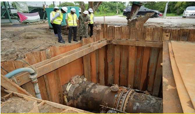
APRIL 2025 SWSI: "GREEN LIGHT" FOR 23 WATER WORKS PROJECTS © PBAPP 2025 Replacement of a faulty 1.2m valve at a pipeline in Jalan Pengkalan Tambang, near the Sungai Dua WTP in SPU.
