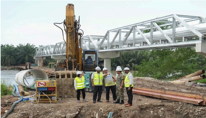
APRIL 2025 SWSI: "GREEN LIGHT" FOR 23 WATER WORKS PROJECTS © PBAPP 2025 Final connection works for the 1.35m Sungai Perai River Crossing Pipeline in Seberang Perai Tengah.
