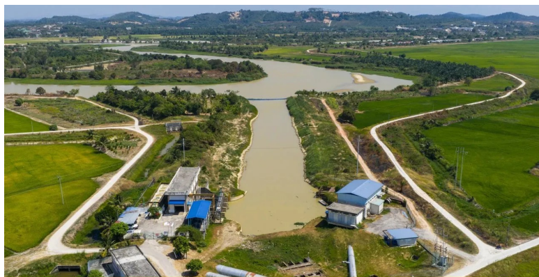
The river level at PBAPP's Lahar Tiang Intake in Seberang Perai Utara (SPU) dipped below the 2.0m mark for 19 consecutive days in January 2026. © PBAPP 2026
