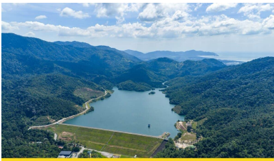
THE MINISTRY OF ENERGY TRANSITION AND WATER TRANSFORMATION (PETRA) PROJECTS FOR PENANG. Water intake works at the Kerawang and Teluk Awak in Teluk Bahang. Including laying a new pipeline from Teluk Kerawang to the Teluk Bahang Dam. © PBAPP 2025
