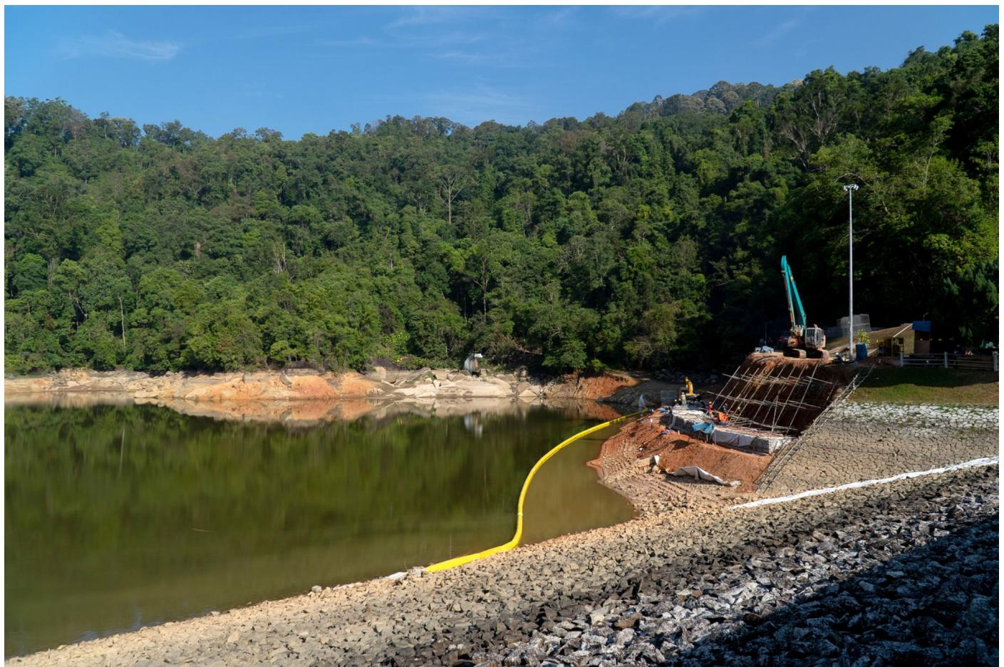
**22.3.2019: Air Itam Dam abutment repair and stabilisation works.**
