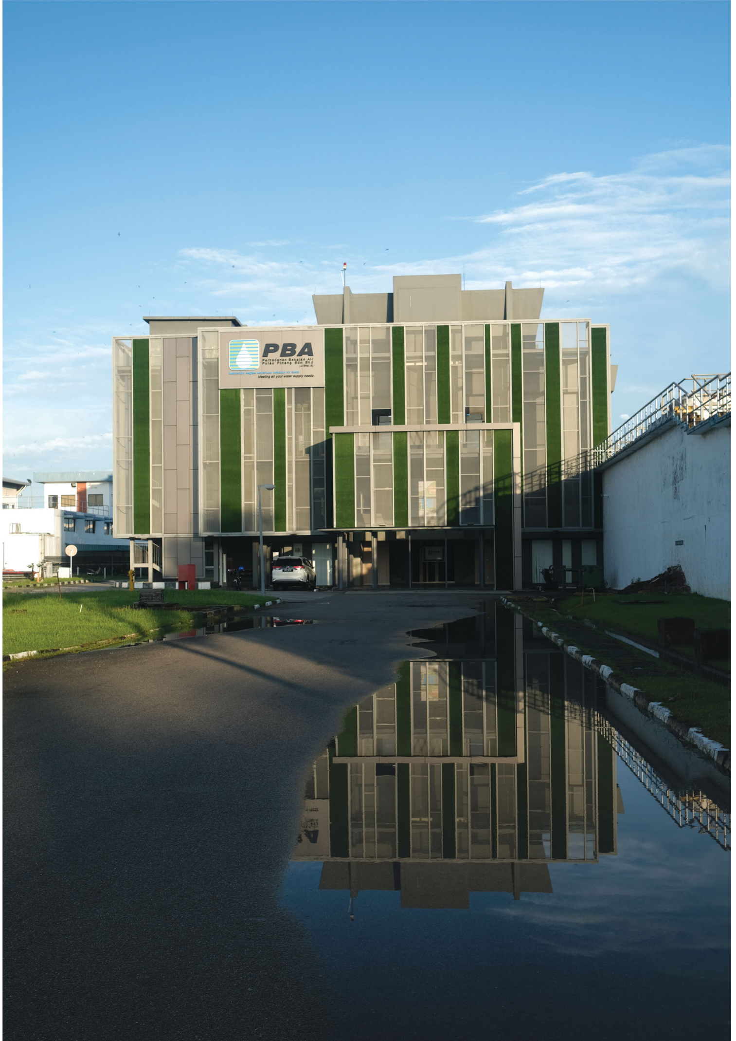
PBAPP's new administration centre, Sungai Dua WTP.
