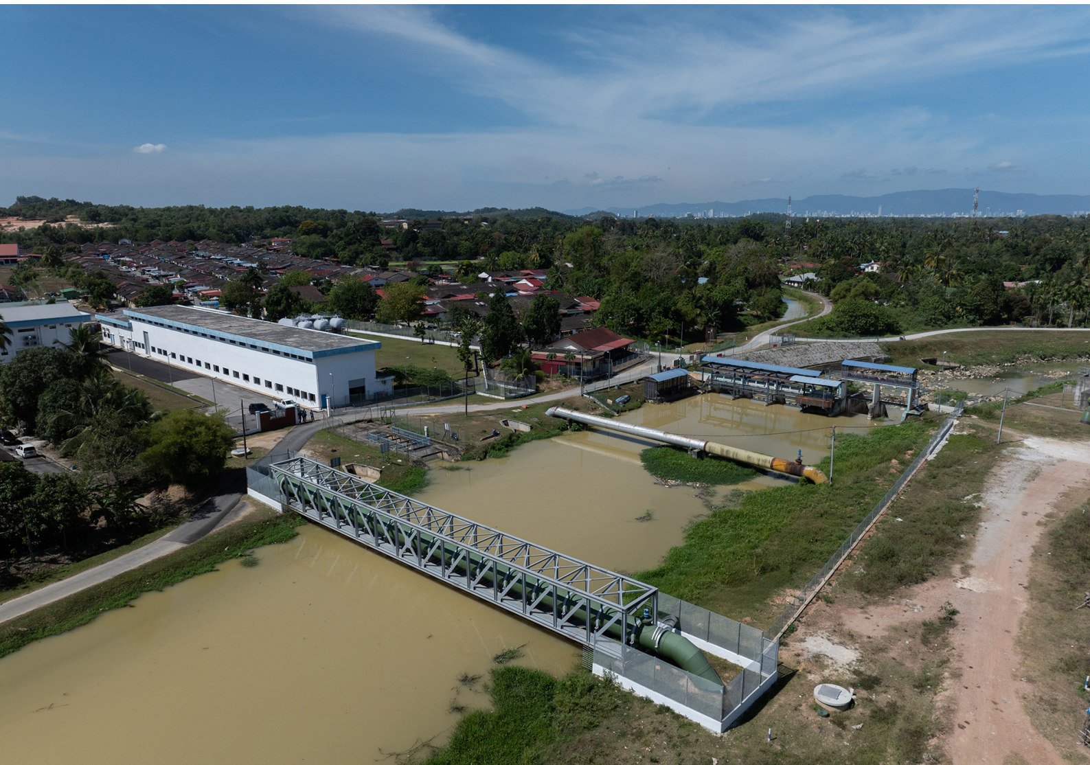
15.2.2024 : PHASE 2B, MENGKUANG DAM EXPANSION PROJECT: ADDITIONAL 300 MLD DRAWDOWN PIPELINE.
